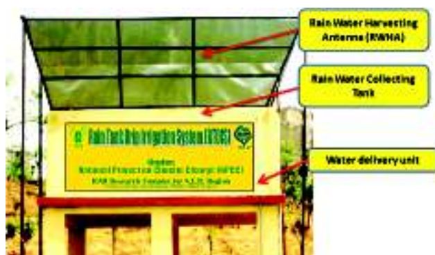
Fig 4 Water Harvesting Antenna and Rain tank unit of Rain Tank Drip Irrigation System (RTDIS)
