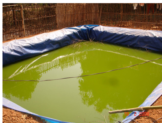
Silpaulin lined Jalkund filled with rain water
