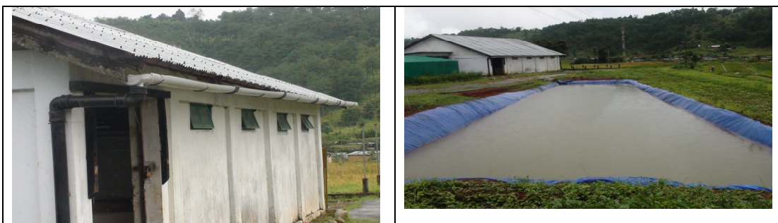
Roof water harvesting in silpaulin lined pond at ICAR, Umiam, Meghalaya..
