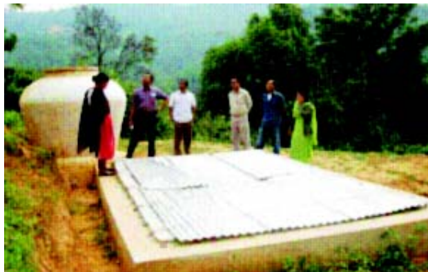
Fig. 27: Jars and ferro-cement lined tanks for intermediate water storage, and is an important element of MUS
