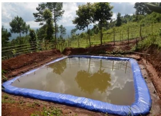
Figure 24: Jalkund constructed at the farmers field in Mawthei village
