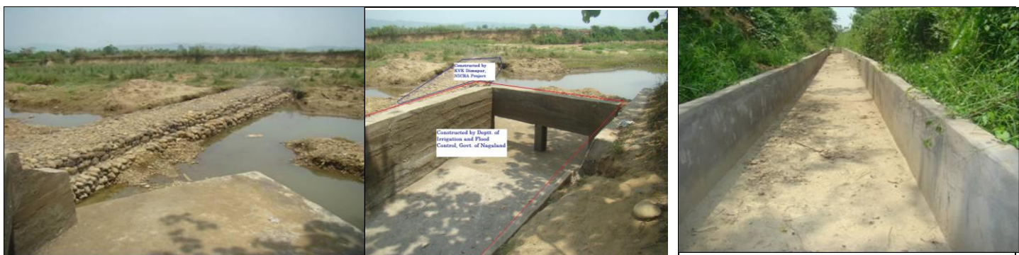
Dam constructed with Sausage wire & boulders
