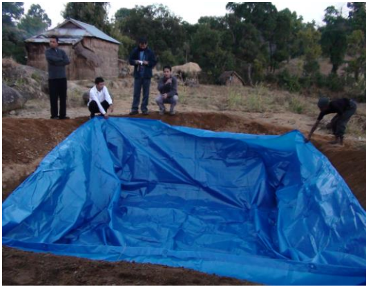
Jalkund with silapaulin lining
