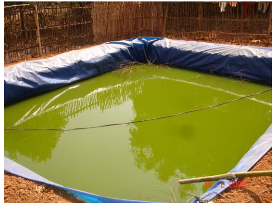
Silapaulin lined Jalkund filled with rain water
